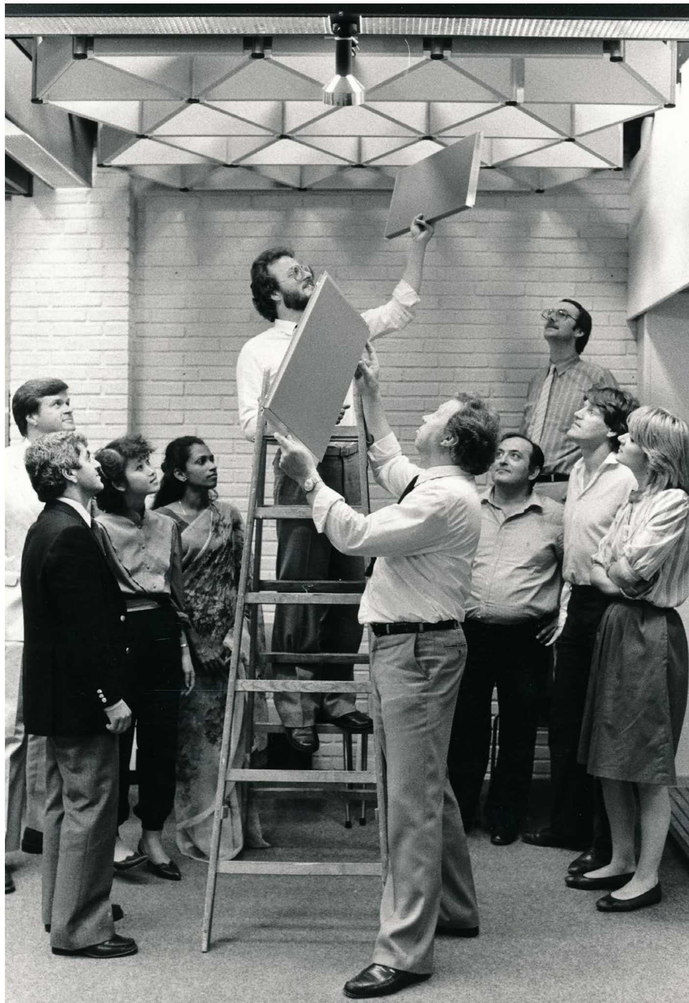
Demonstration of installation of DAMPA Baffler, cirka 1983
